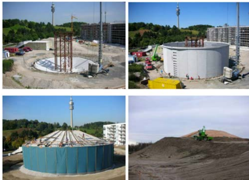
Figure 1.2 Construction of a tank thermal energy storage system in Munich, Germany [17]
